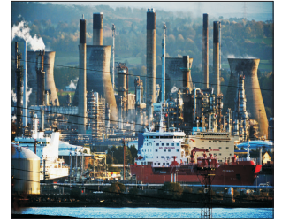
Refinery Petrochemical Plant
